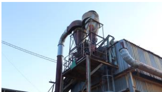
Fuel House Cyclone #SLM_DM_65
